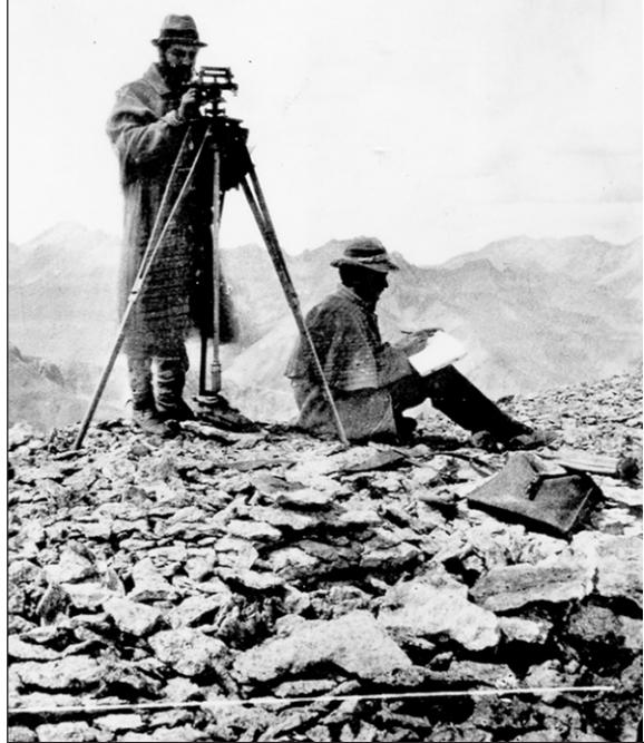
Hayden Survey topographers Allen D. Wilson, with transit, and Franklin Rhode, seated with field notebook, were memorialized in an 1874 photo by W.H. Jackson on the summit of Sultan Mountain in 1874; the photo was in turn used as the basis for a steel engraving for publishing purposes. — U.S. Geological Survey
